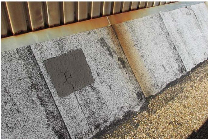
*Worn and patched roof flashing; rusting at roof screen*
