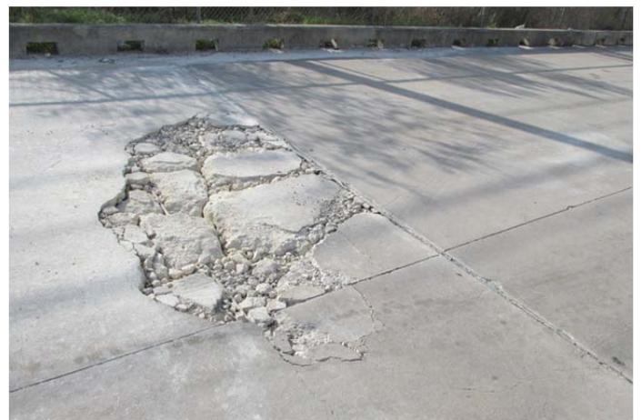
*Severely distressed concrete pavement*
