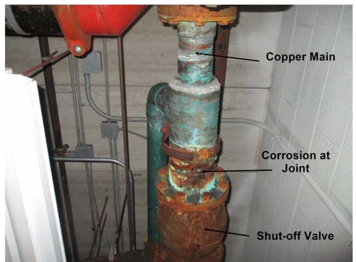
*Rusting and deterioration of piping critical to the building's operation*
